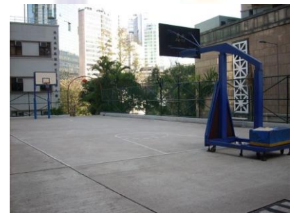
Outdoor School Playground
